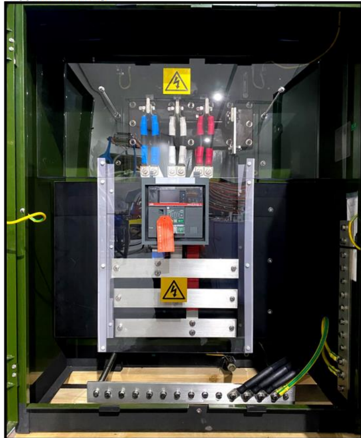
1600 AMP ABB ACB WITH FLEXIBLE INCOMERS
